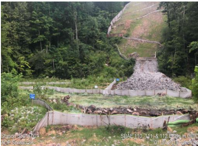
Spread 2A – Stabilized ROW / ECD inspection
