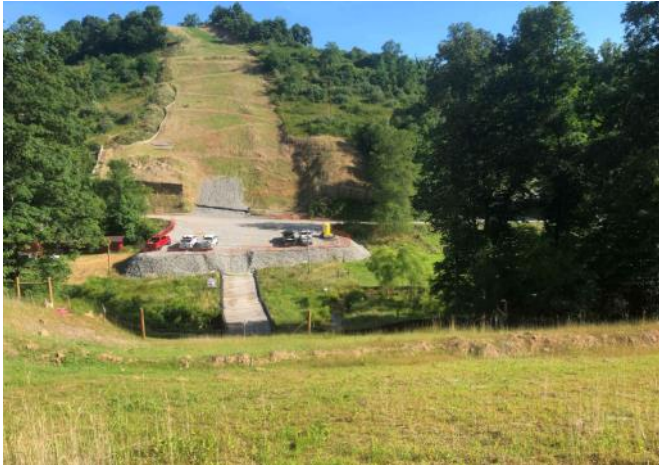
Spread 1-1 – Stabilized ROW
