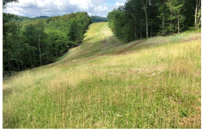
Spread 1-2 – Stabilized ROW
