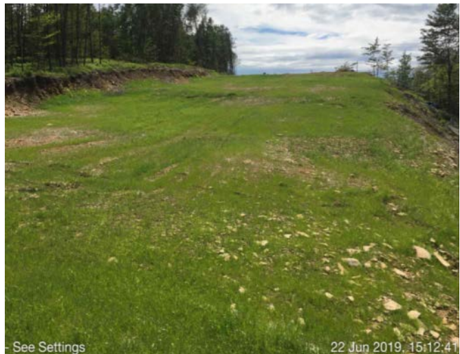
Spread 2-2 – Stabilized ROW
