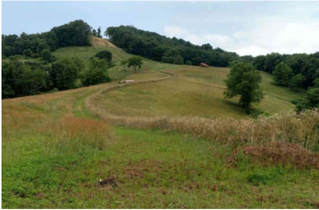
Spread 1-1 – Stabilized ROW
