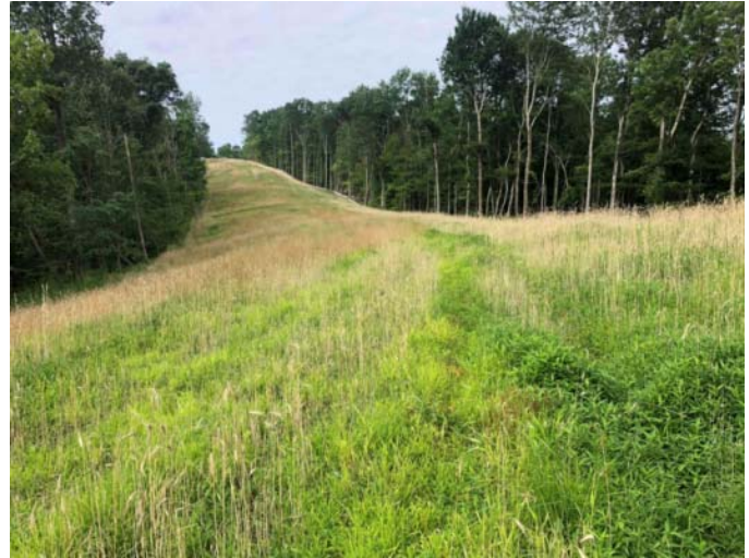
Spread 1-2 – Stabilized ROW
