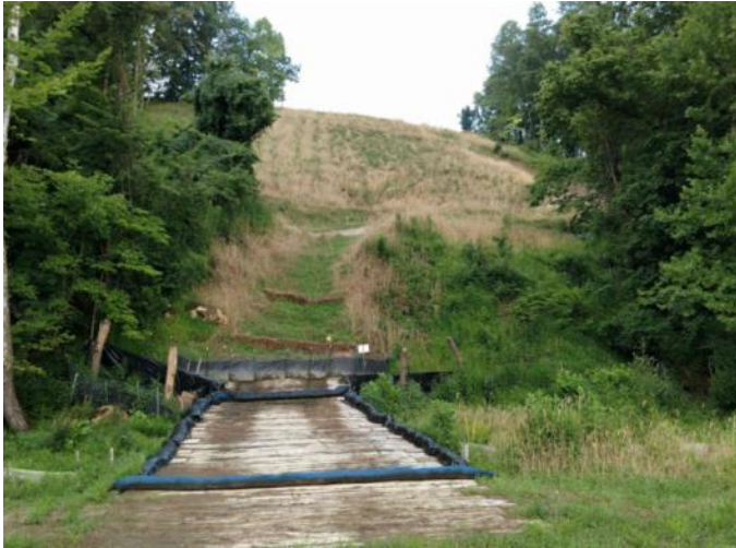
Spread 1-1 – Stabilized ROW
