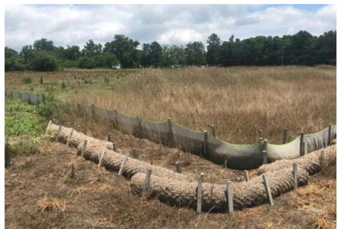
Spread 10 – Stabilized ROW
