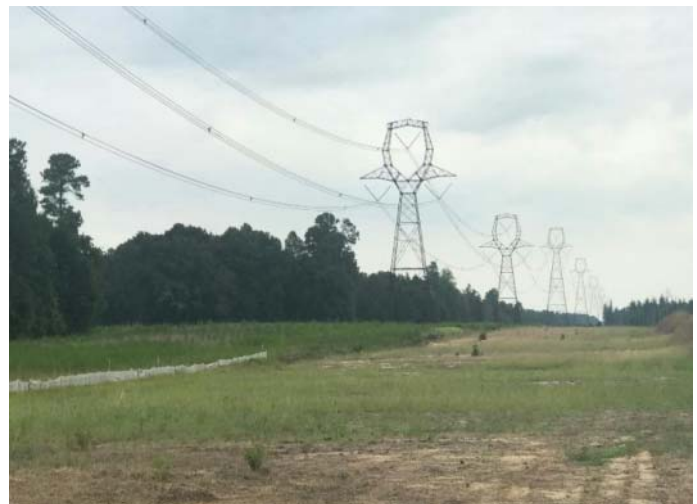
Spread 10 – Stabilized ROW
