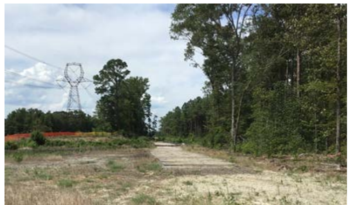
Spread 10 – Stabilized ROW
