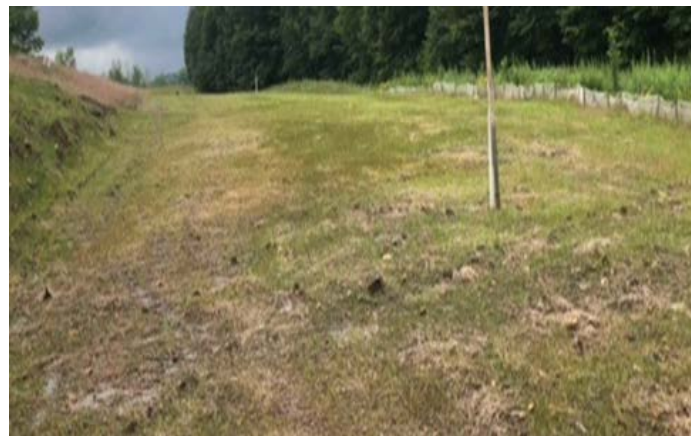
Spread 2A – Stabilized ROW
