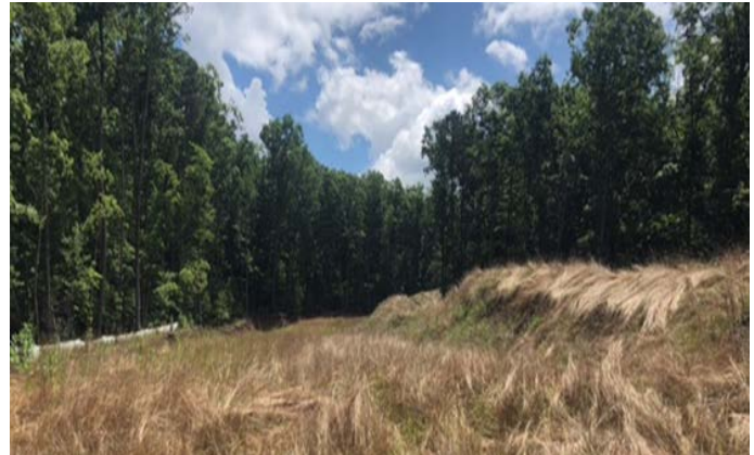
Spread 3 – Stabilized ROW
