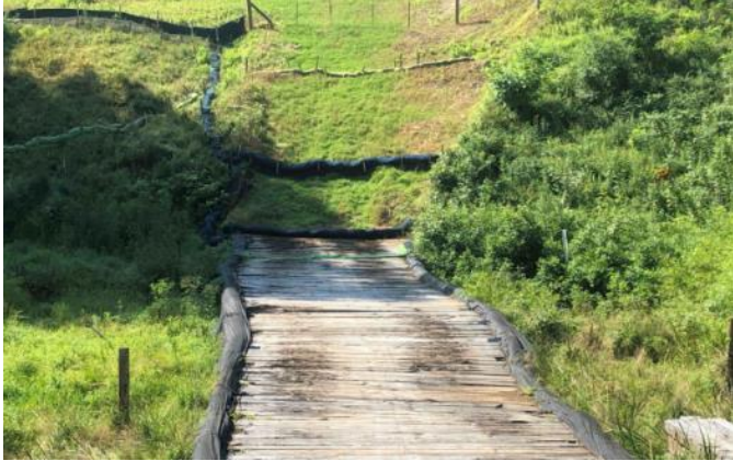
Spread 1-1 – Stabilized ROW
