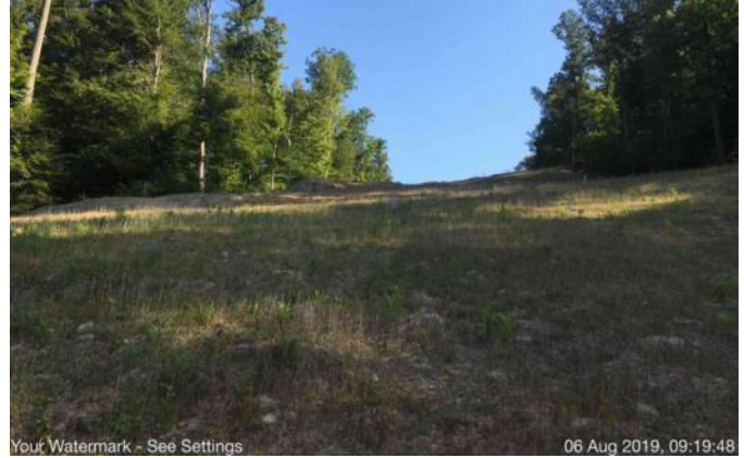
Spread 2-1 – Stabilized ROW
