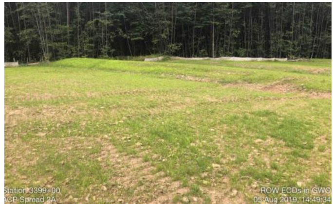
Spread 2A – Stabilized ROW
