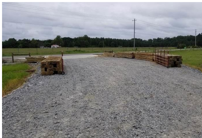
Spread 8 – Halifax Yard Gate Installation
