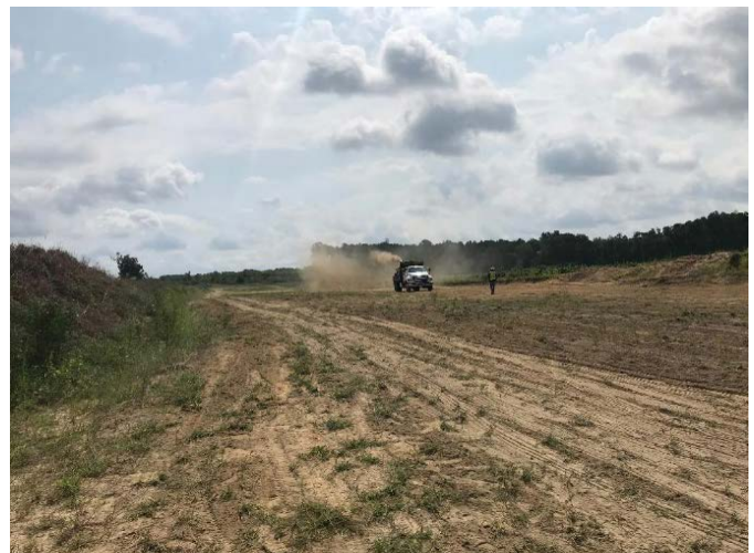
Spread 10 – Reseeding and Mulching ROW
