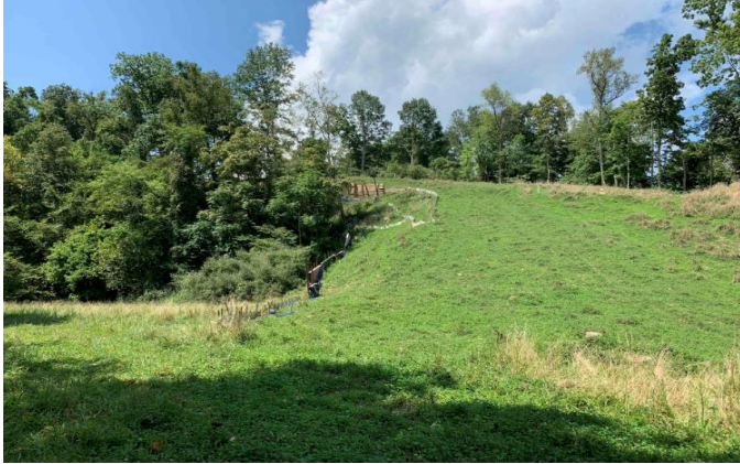
Spread 1-1 – Stabilized ROW
