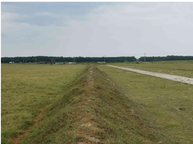
Spread 8 – Stabilized topsoil pile
