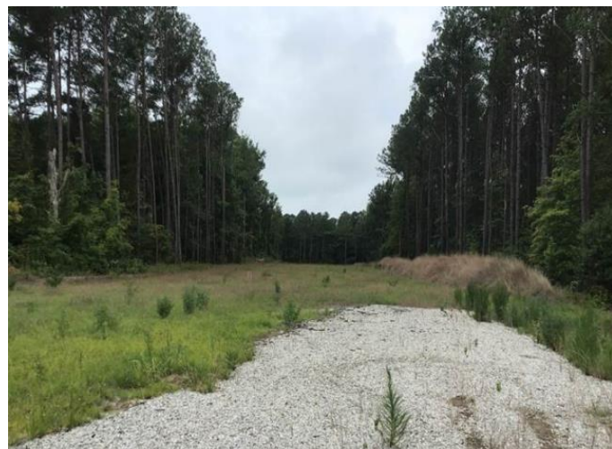
Spread 10 – Stabilized ROW
