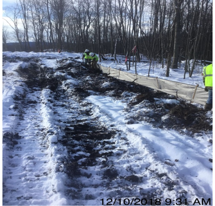
Spread 2A Installing silt fence
