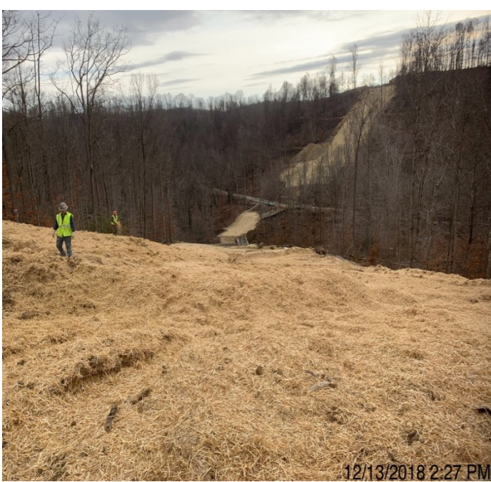
Spread 2-1 Hand mulching the ROW
