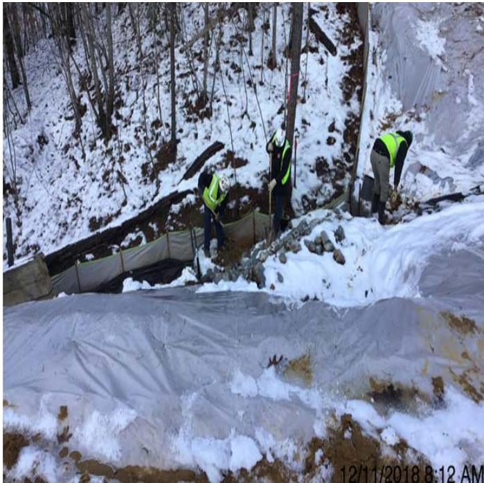
Spread 8 Repairing silt fence
