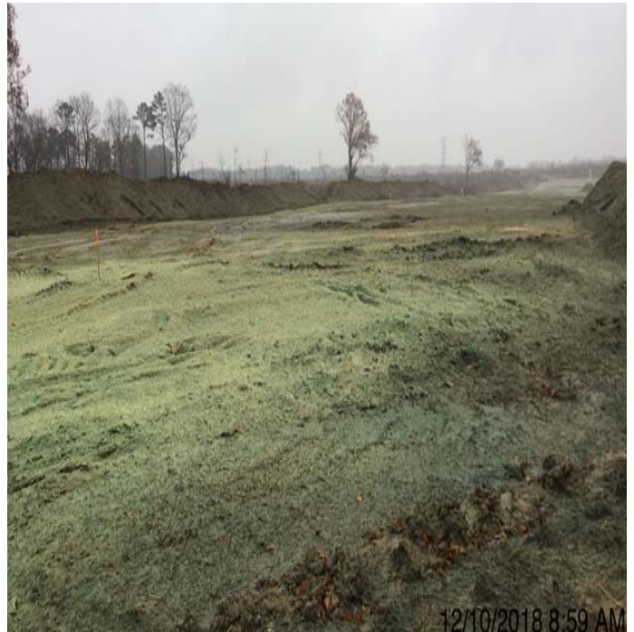
Spread 10 Hydro-mulched ROW for stabilization
