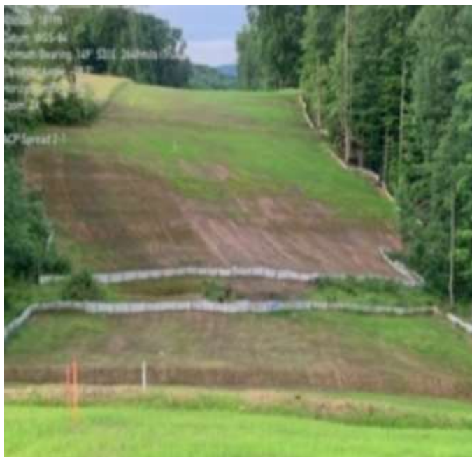
Spread 2-1 – Stabilized ROW
