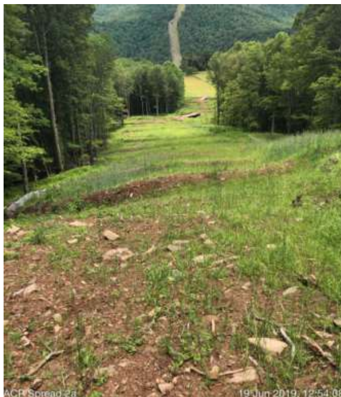
Spread 2A – Stabilized ROW
