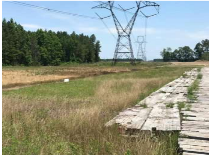
Spread 10 – Stabilized ROW
