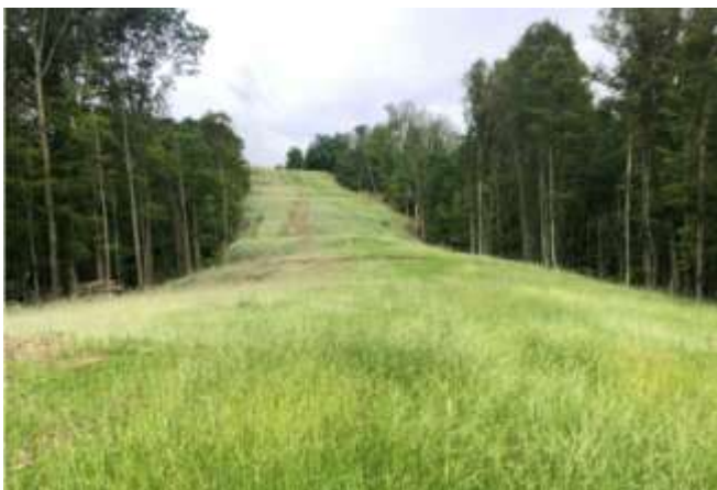
Spread 1-2 – Stabilized ROW
