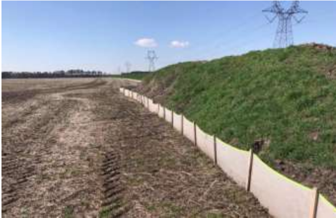
Spread 10 – Stabilized ROW
