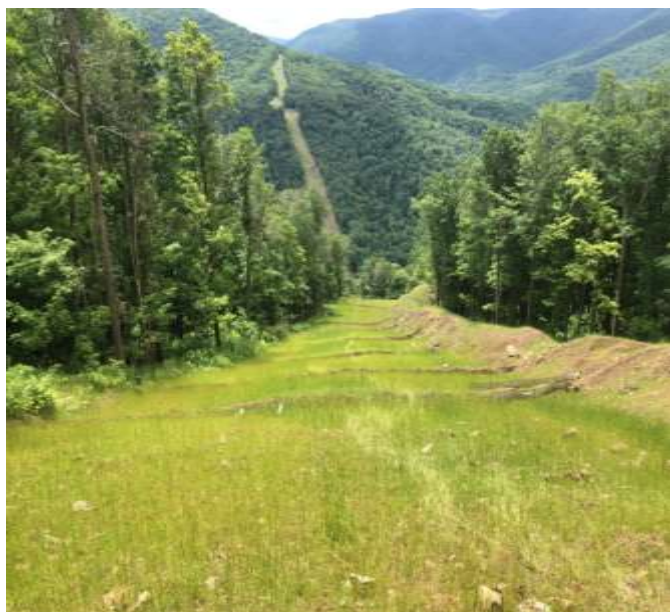
Spread 2A – Stabilized ROW
