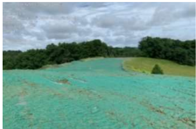
Spread 2-1 – Hydroseeded ROW
