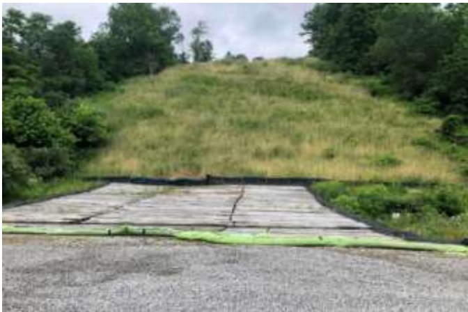
Spread 1-1 – Stabilized ROW
