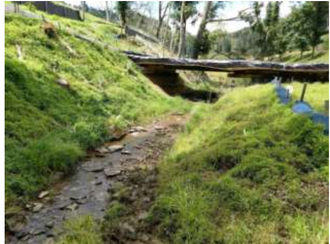
Spread 1-1 – Stream & ECD inspection
