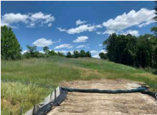
Spread 1-1 – Stabilized ROW
