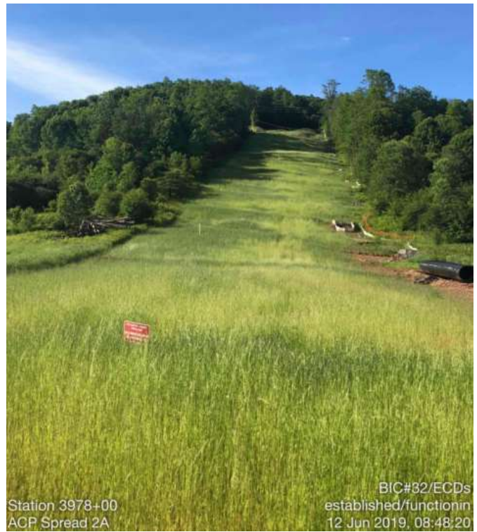
Spread 2A – Stabilized ROW
