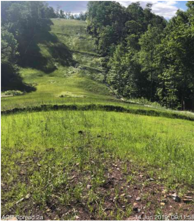
Spread 2A – Stabilized ROW
