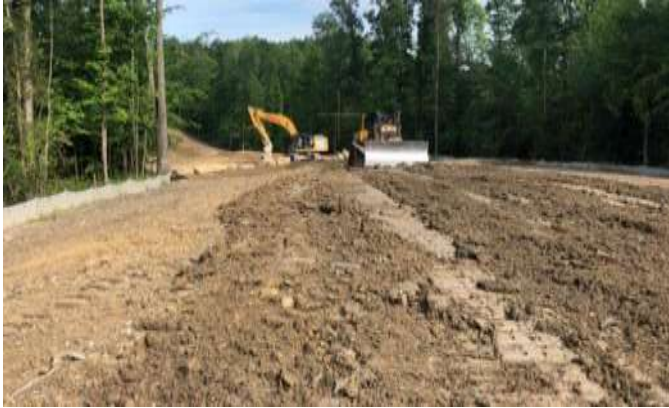
Spread 2-1 – Restoring grade
