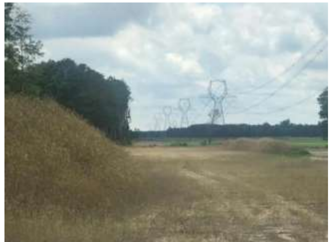
Spread 10 – Stabilized ROW
