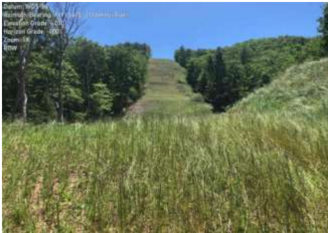
Spread 3A – Stabilized ROW
