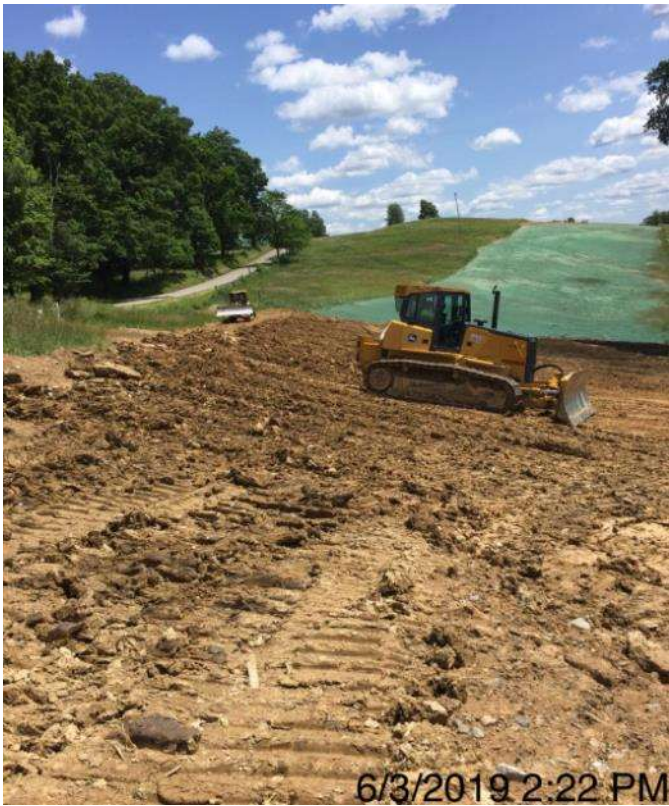
6/3/2019 2:22 PM Spread 2-1 – Restoring grade
