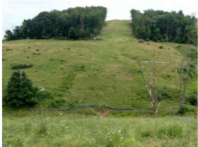
Spread 1-1 – Stabilized ROW
