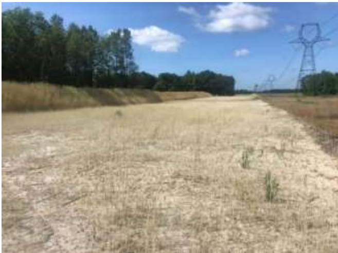
Spread 10 – Stabilized ROW
