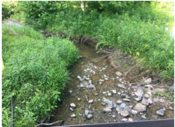
Spread 1-1 – Stream inspection
