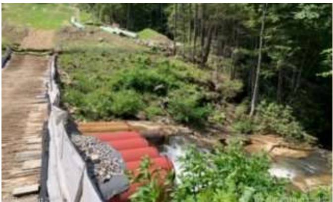
Spread 2-1 – Stream inspection
