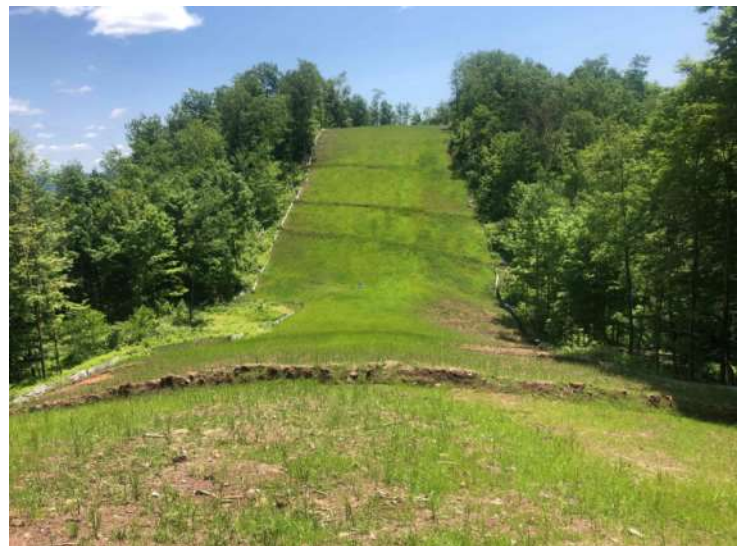
Spread 2A – Stabilized ROW
