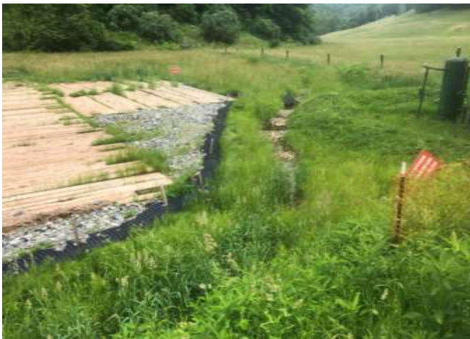
Spread 1-2 – Stabilized ROW
