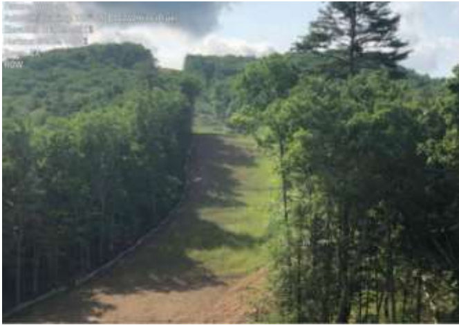
Spread 3A – Stabilized ROW
