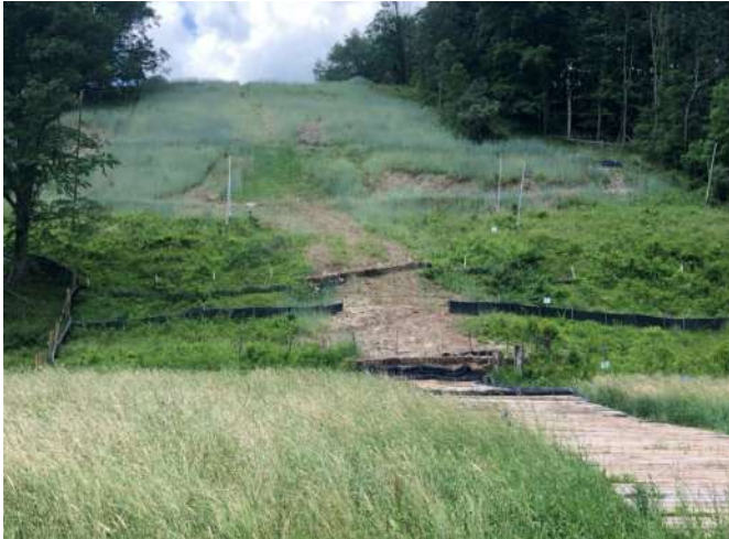
Spread 1-1 – Stabilized ROW
