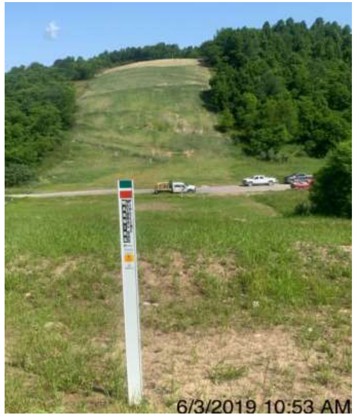
6/3/2019 10:53 AM Spread 2-1 – Fully restored ROW
