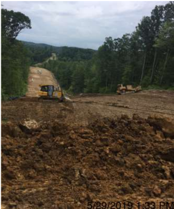
Spread 2-1 – Installing waterbar
