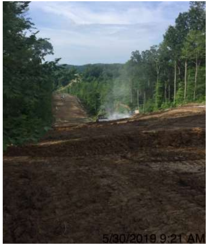
Spread 2-1 – Drying soil with lime
