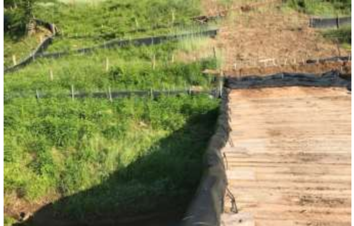
Spread 1-2 – ECD inspection
