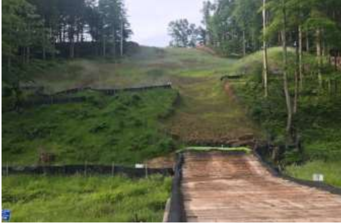
Spread 1-1 – Stabilized ROW
