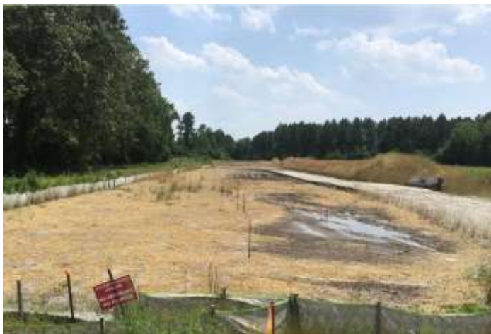
Spread 10 – Stabilized ROW
