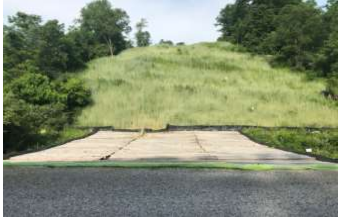
Spread 1-1 – Stabilized ROW
