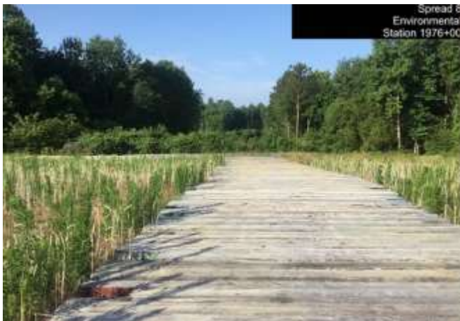
Spread 8 – Stabilized ROW
