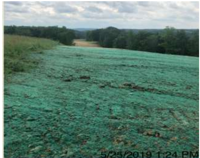
Spread 2-1 – Hydroseeded ROW
