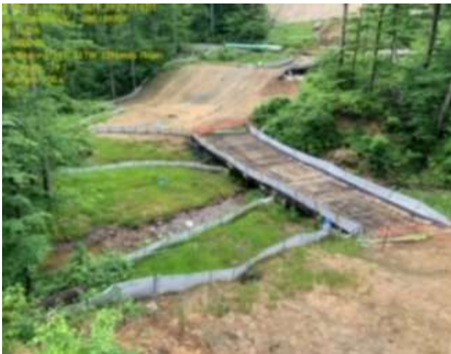
Spread 2-1 – ECD inspection
