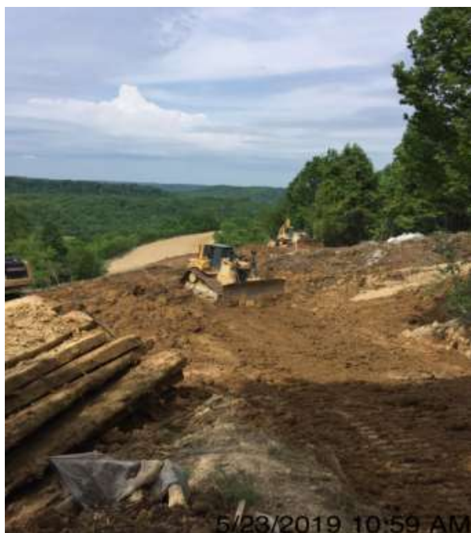
Spread 2-1 – Restoring grade
