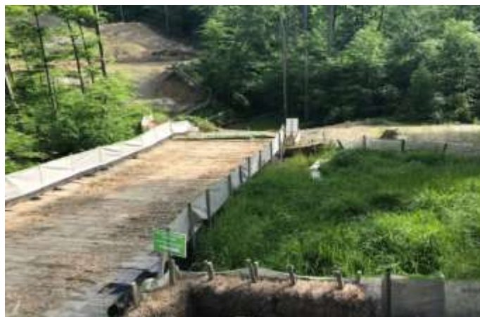
Spread 2-1 – ECD inspection at stabilized stream
