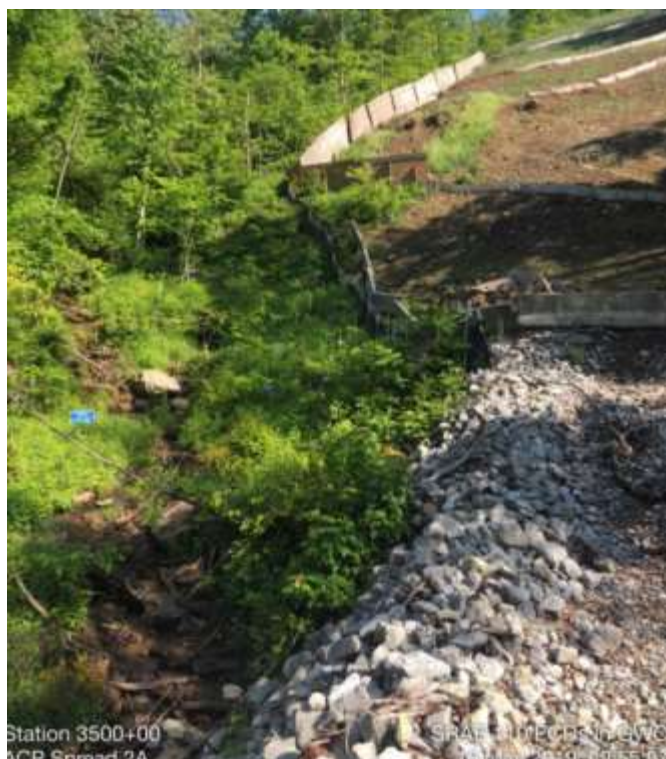
Spread 2A – Inspecting ECDs
