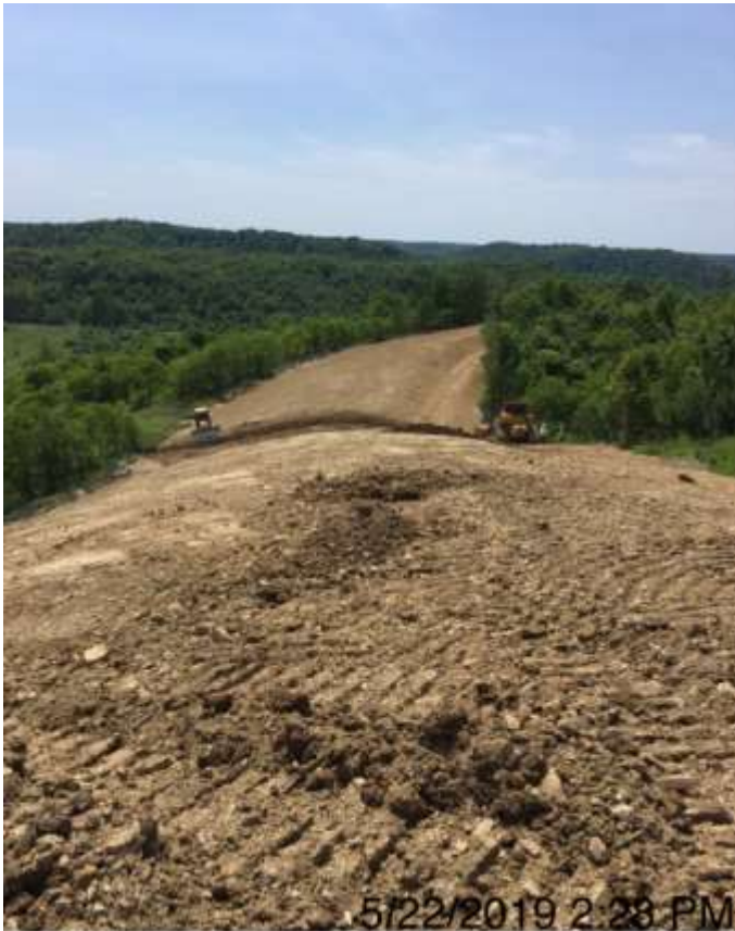
Spread 2-1 – Installing waterbar
