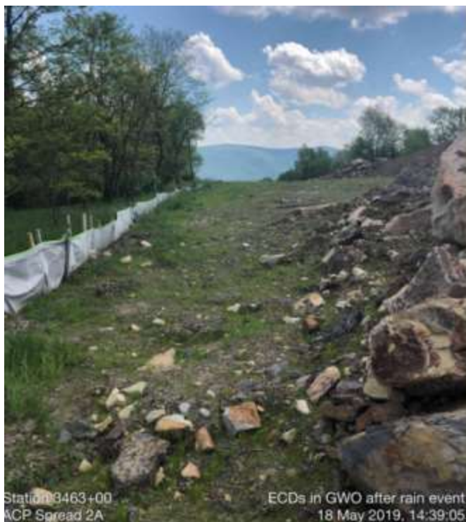
Spread 2A – Stabilized ROW
