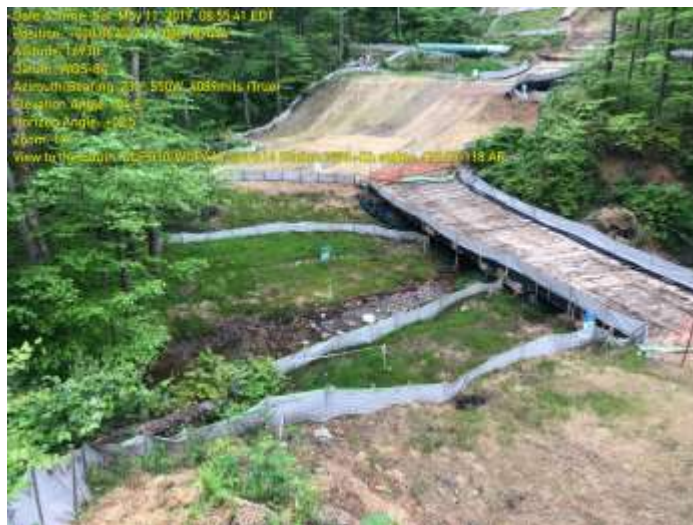
Spread 2-1 – ECD Inspection
