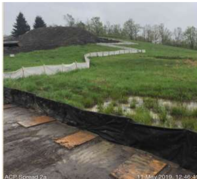
Spread 2A – Inspecting ECDs
