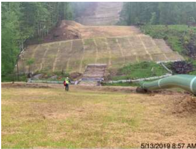
Spread 2-1 Hand seeding over sparsely covered areas
