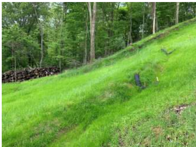
Spread 1-1 – Stabilized ROW
