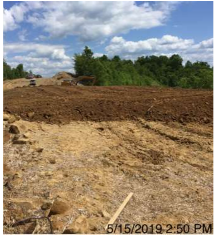
Spread 2-1 – Restoring grade
