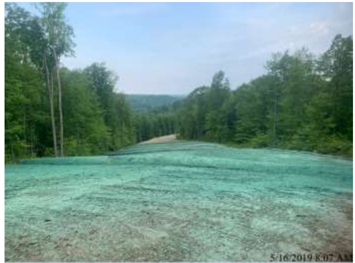
Spread 2-1 – Hydroseeded ROW
