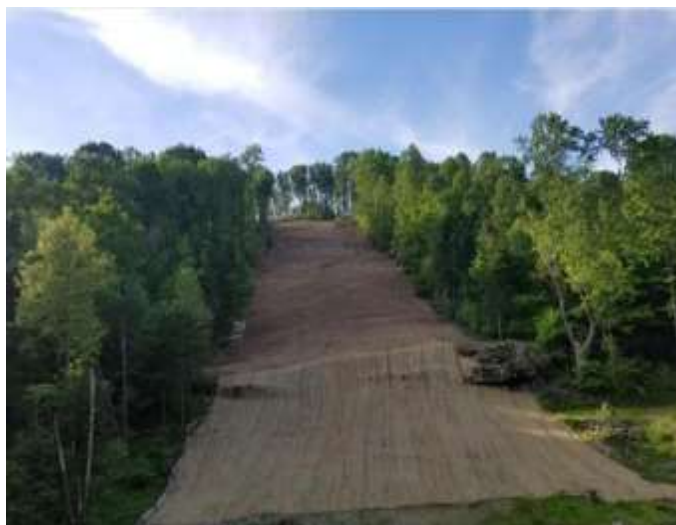
Spread 2-1 – Stabilized ROW
