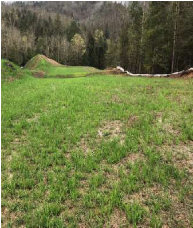
Spread 3A – Stabilized ROW
