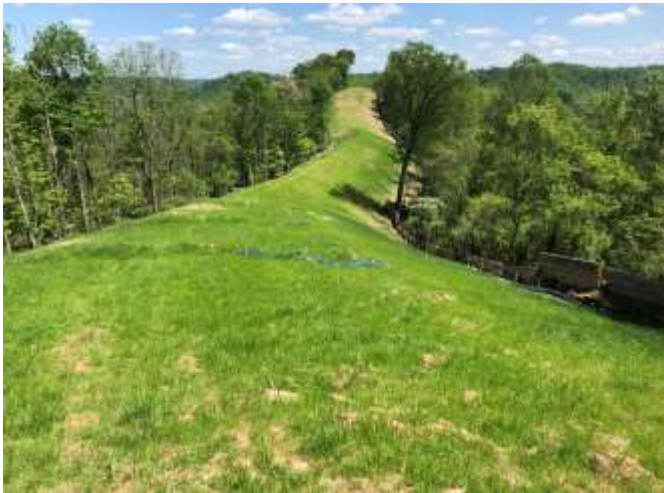
Spread 1-1 – Stabilized ROW
