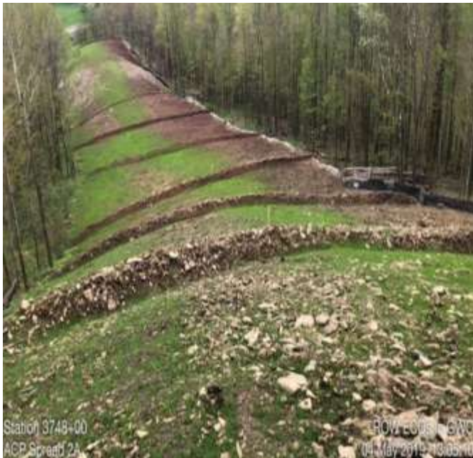
Spread 2A – Stabilized ROW
