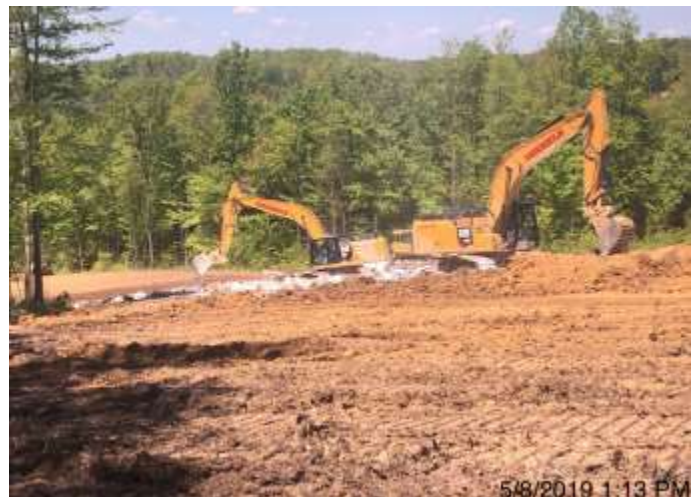
Spread 2-1 – Drying the ROW
