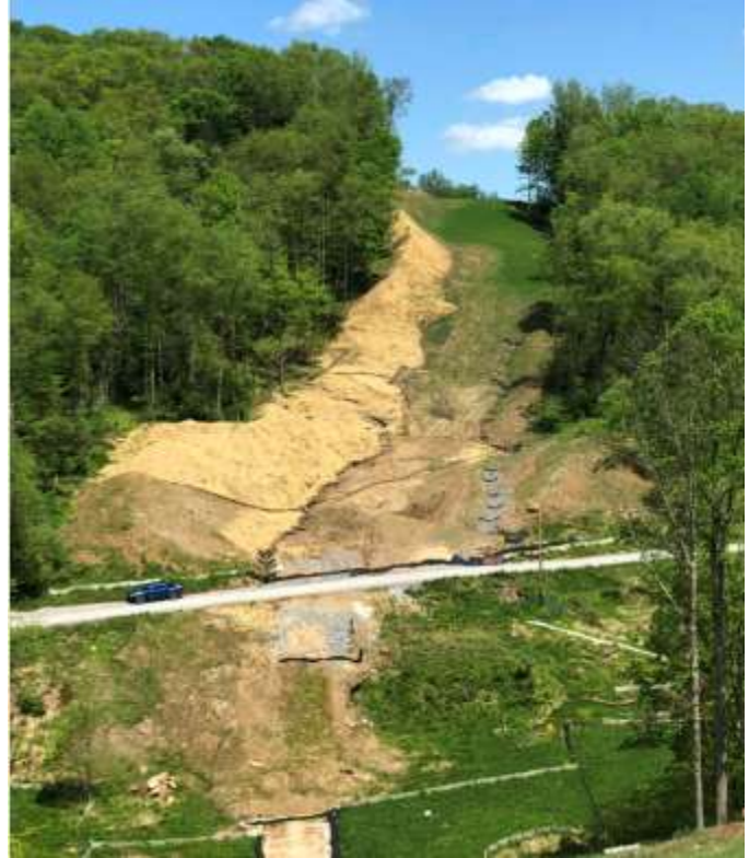
Spread 1-1 – Stabilized ROW
