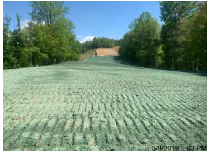
Spread 2-1 – Hydroseeded ROW
