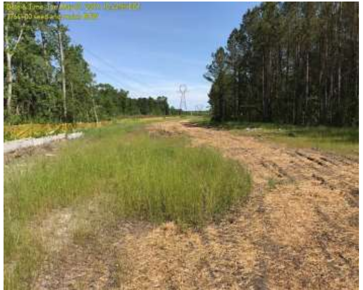
Spread 10 – Stabilized ROW
