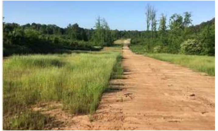
Spread 8 – Stabilized ROW
