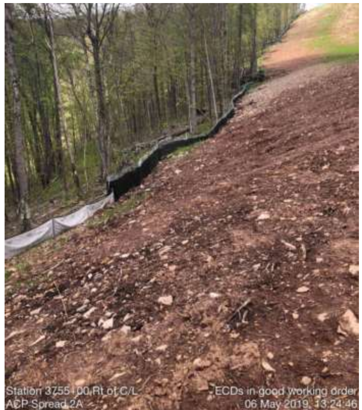
Spread 2A – Inspecting ECDs
