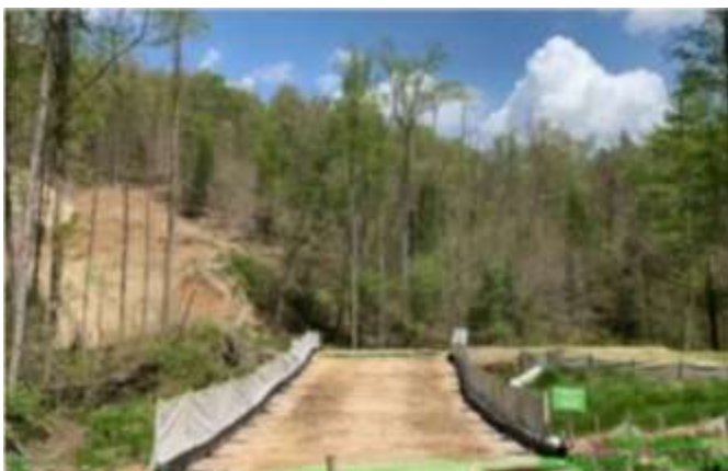
Spread 2-1 – ECD inspection
