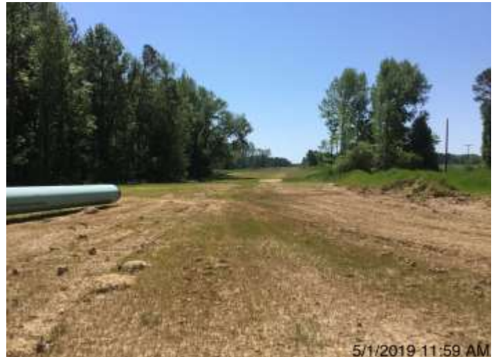
Spread 8 – Stabilized ROW
