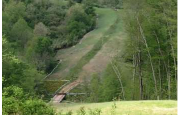
Spread 1-1 – Stabilized ROW
