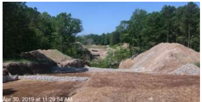
Spread 10 – Stabilized ROW
