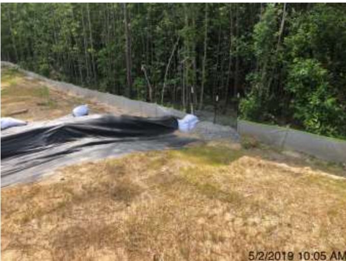
Spread 8 – ECD Inspection
