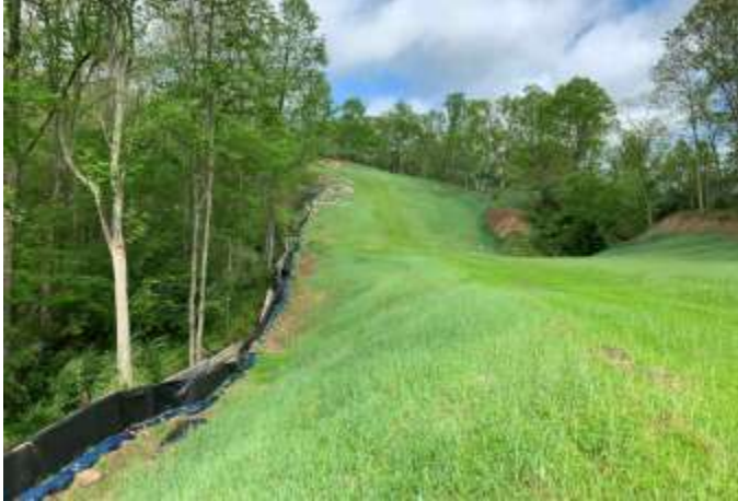
Spread 1-1 – Stabilized ROW
