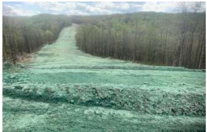
Spread 2-1 – Hydroseeded ROW
