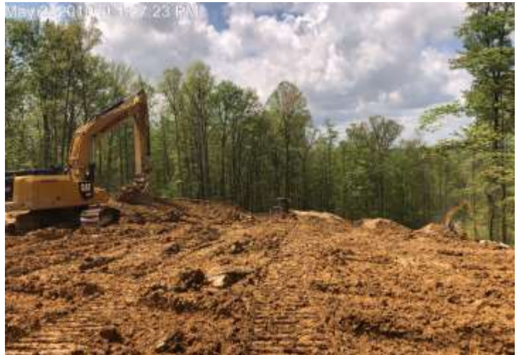
Spread 2-1 – Drying the ROW
