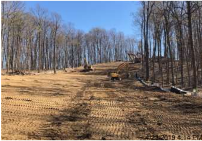
Spread 2-1 – Grading
