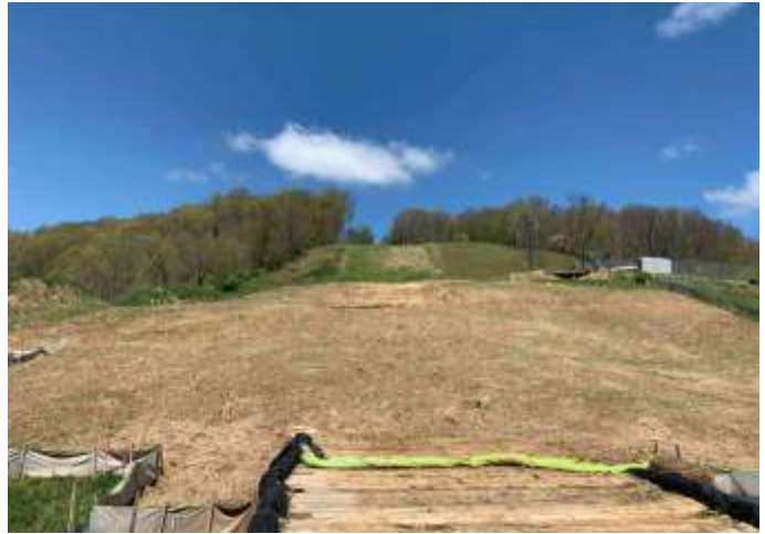
Spread 2-1 – Stabilized ROW
