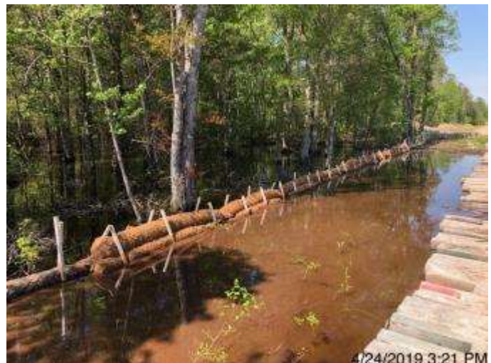
Spread 8 – ECD inspection
