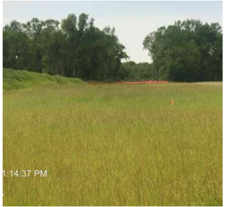
Spread 10 – Stabilized ROW
