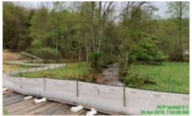
Spread 2-1 – ECD inspection
