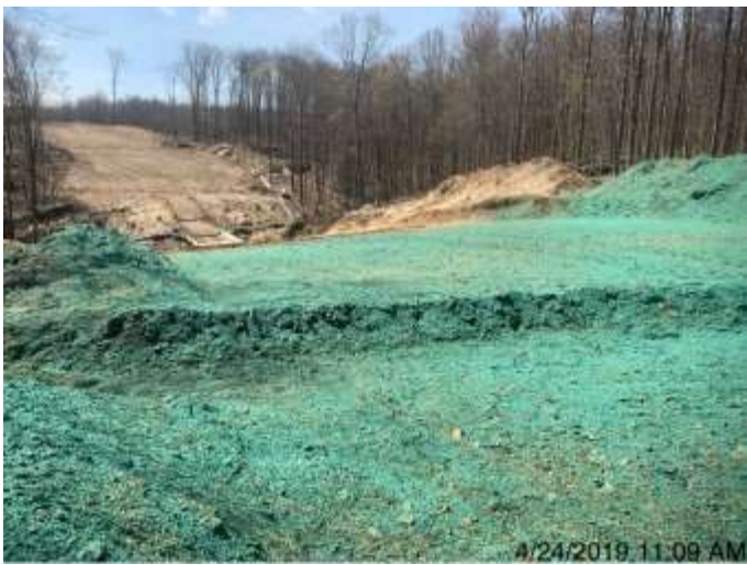
Spread 2A – Stabilized ROW
