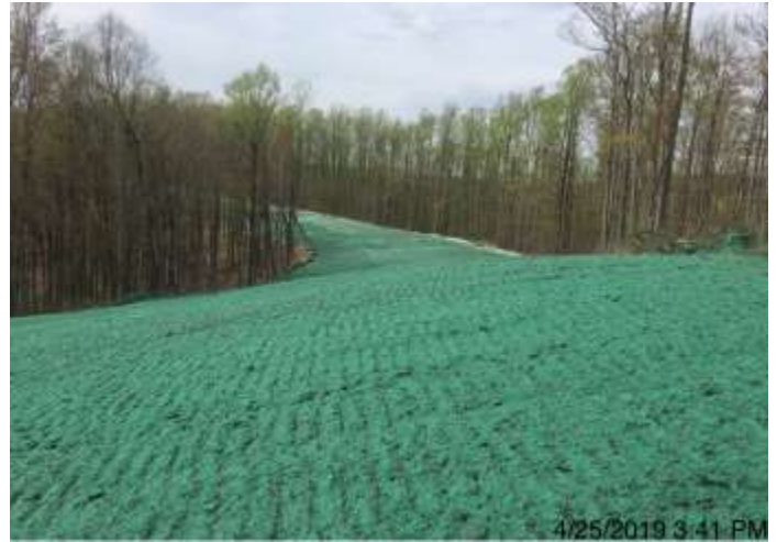
Spread 2-1 – Hydroseeded ROW
