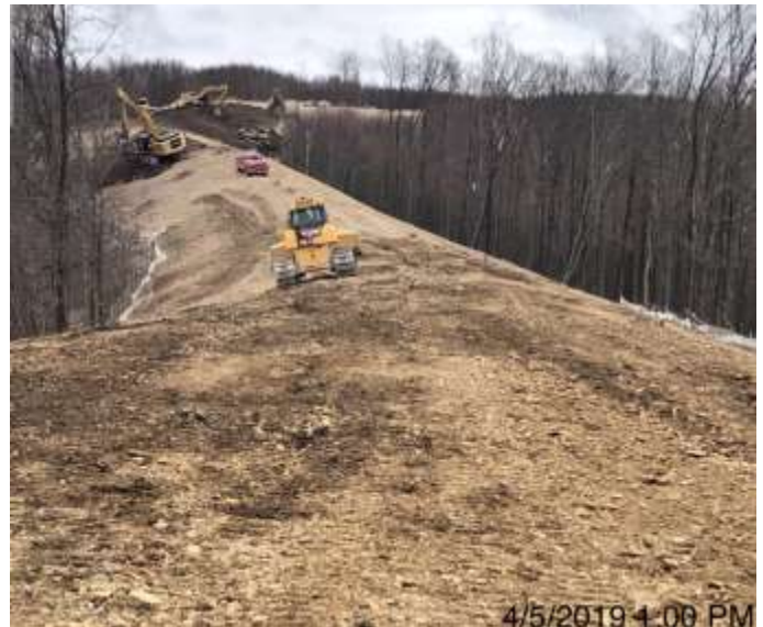
Spread 2-1 – Stabilizing ROW
