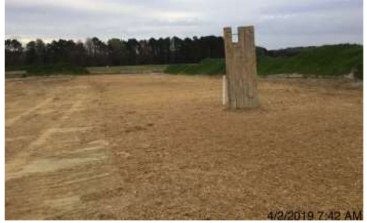
Spread 8 – Tar River drill exit stabilized
