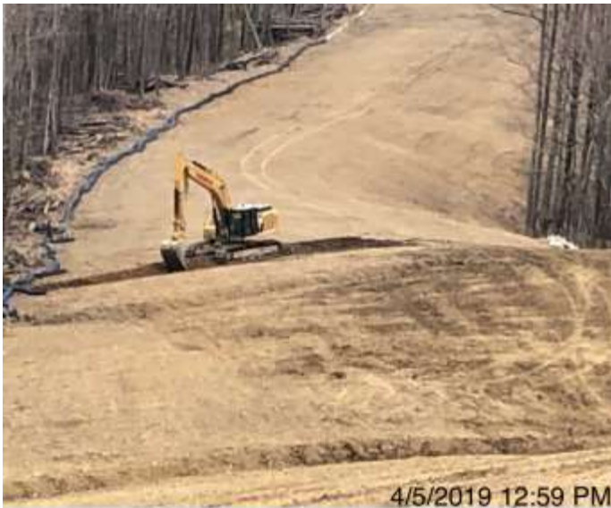
Spread 2-1 – Waterbar installation
