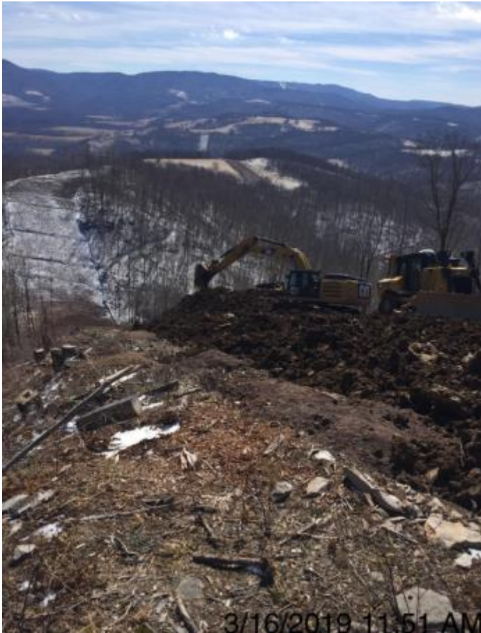
Spread 2A – Restoration on hillside
