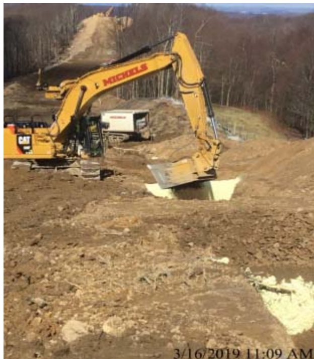
Spread 2-1 – Padding/Backfilling
