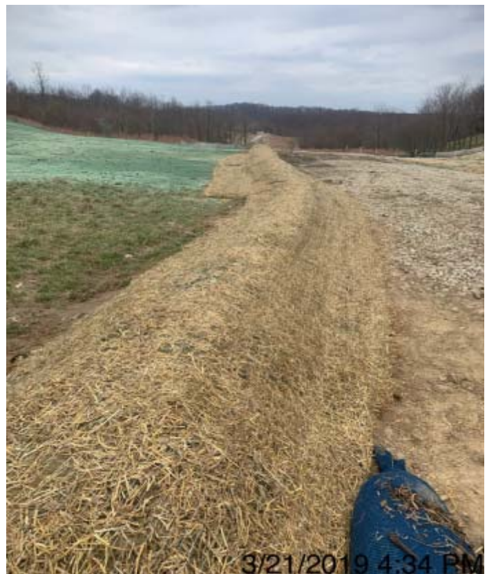
Spread 2-1 – Stabilized ROW
