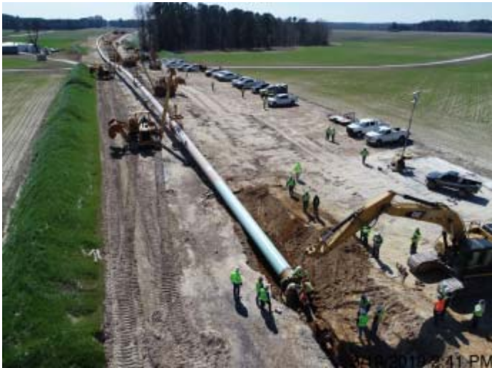
Spread 8 – Pulling section into drill hole
