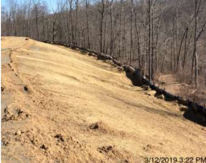
Spread 1-1 – Stabilized ROW
