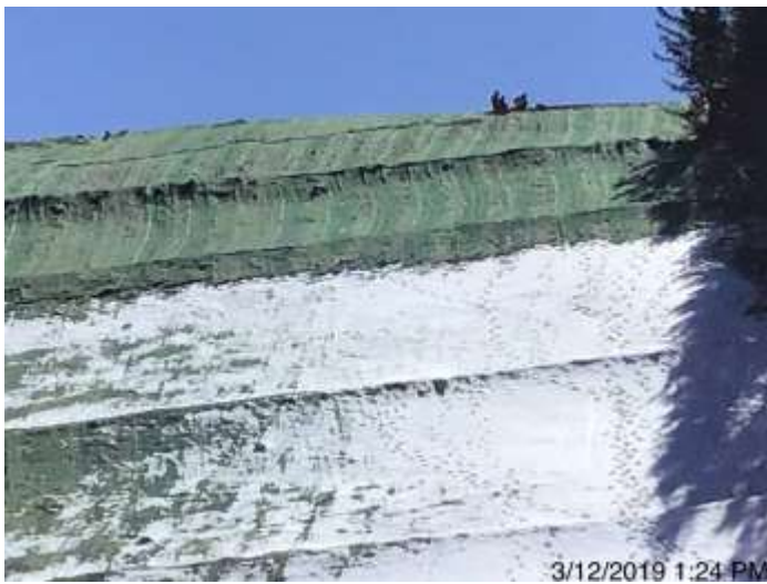
Spread 2A – Curlex on hillside
