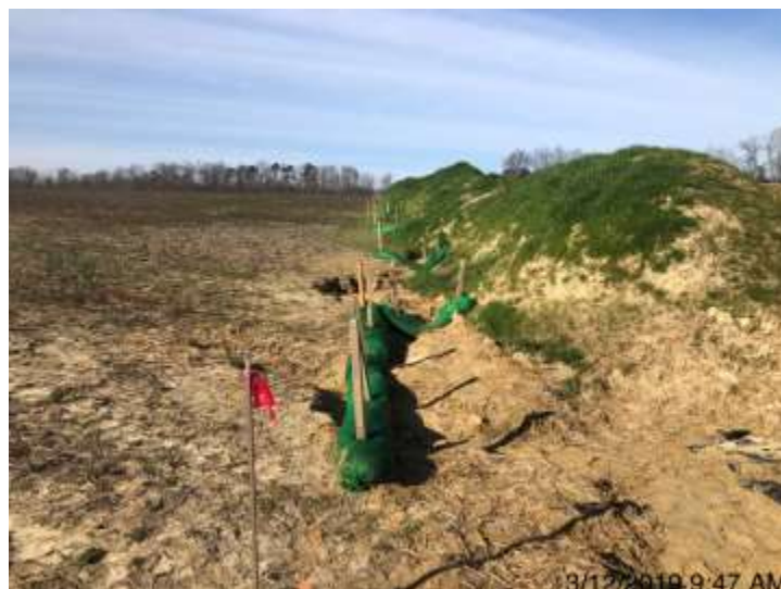
Spread 8 – Stabilized ROW
