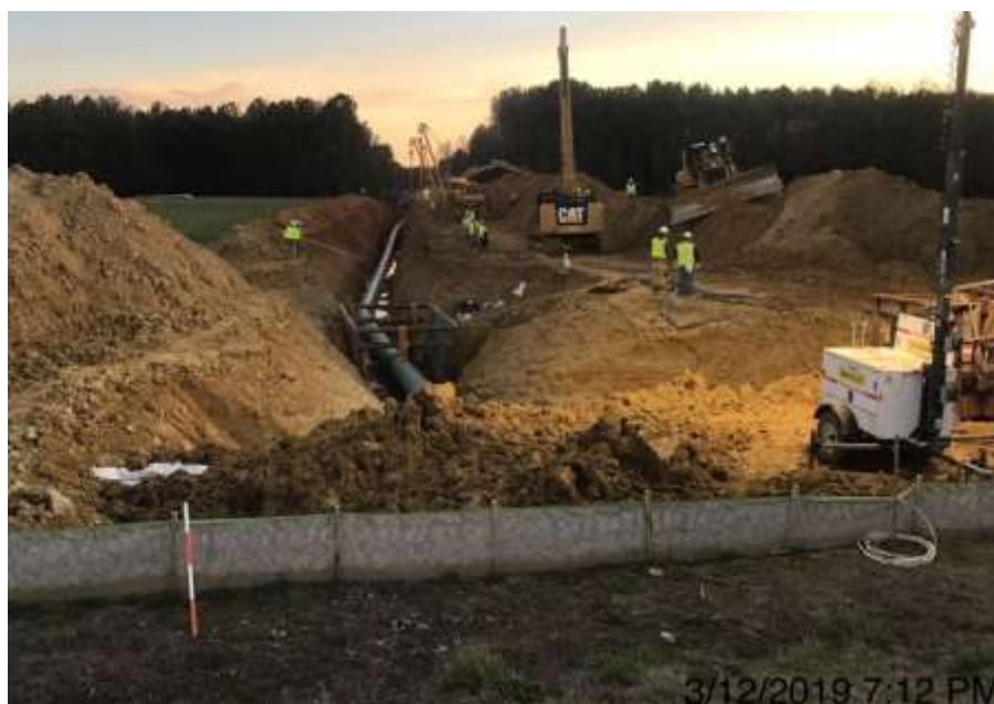
Spread 8 – Tie in weld
