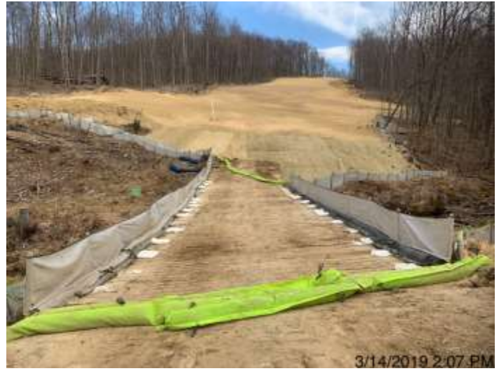
Spread 2-1 – Stabilized ROW
