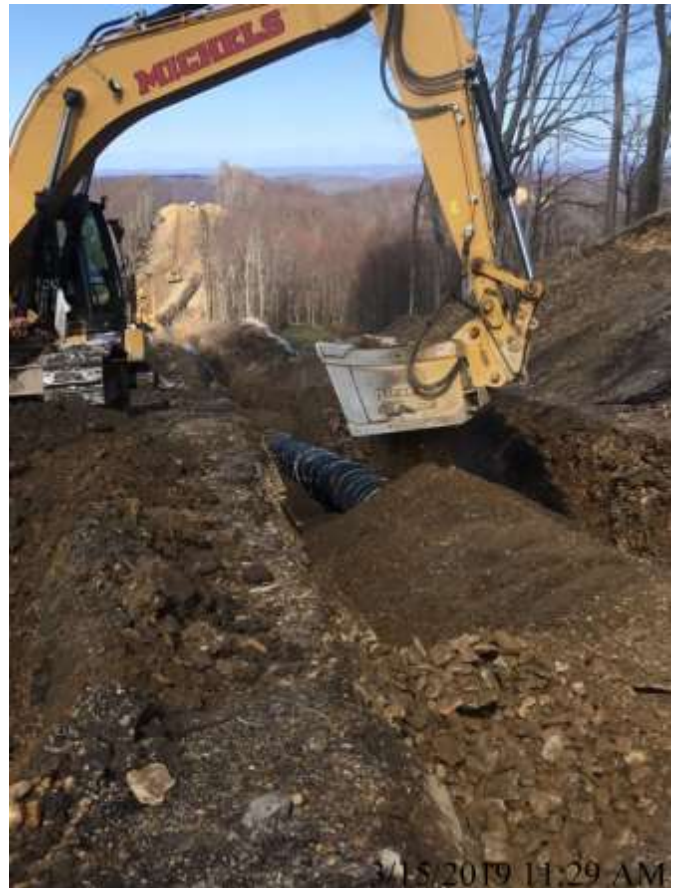
Spread 2-1 – Padding/Backfilling
