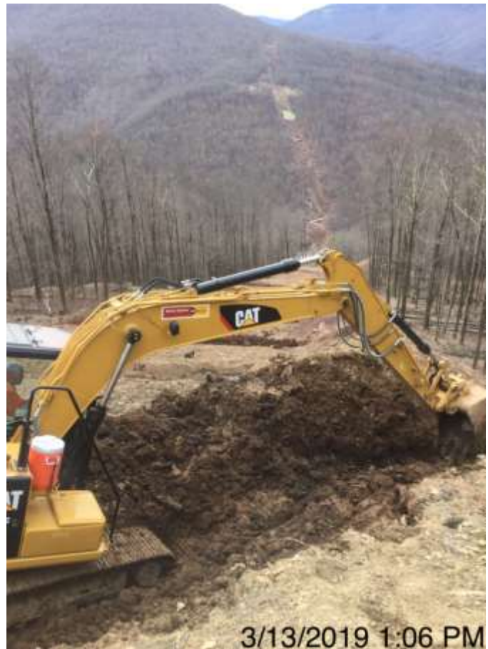
Spread 2A – Clean up and installing water bars
