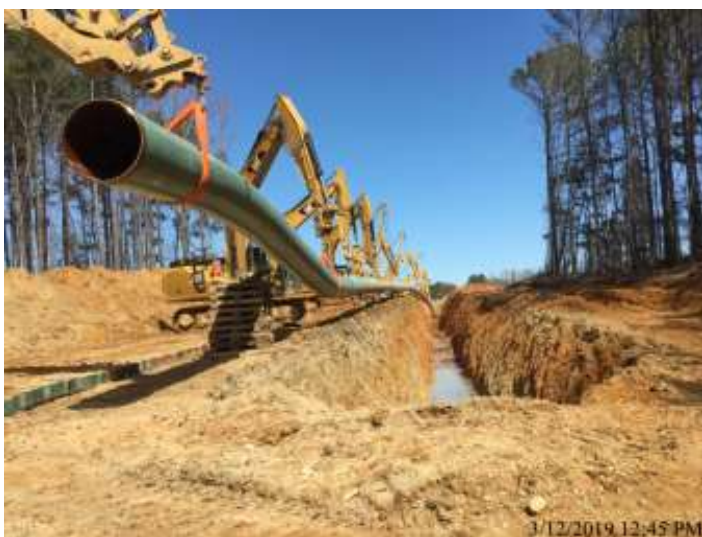
Spread 8 – Prep for lowering in
