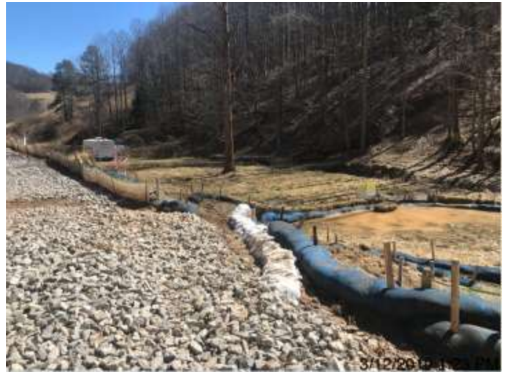
Spread 1-1 – Stabilized ROW
