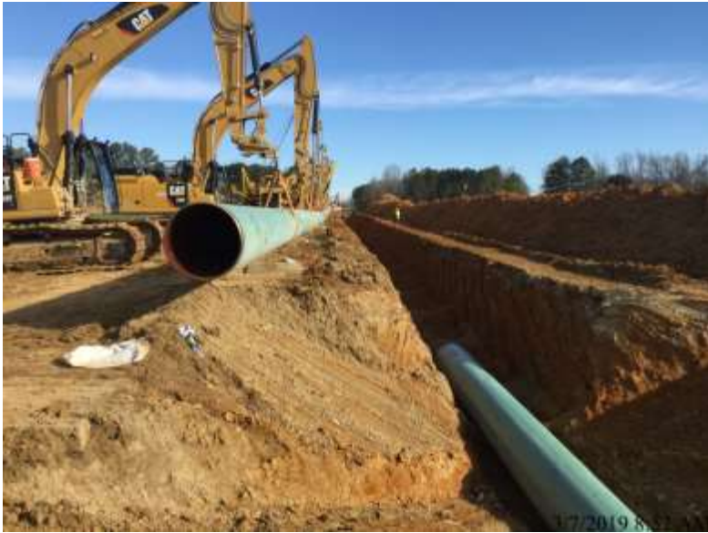
Spread 8 – Prep for lowering in
