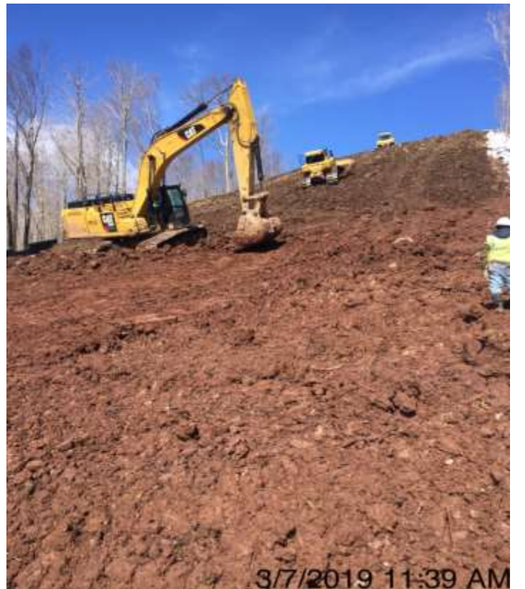
3/7/2019 11:39 AM Spread 2A – Clean up and installing water bars
