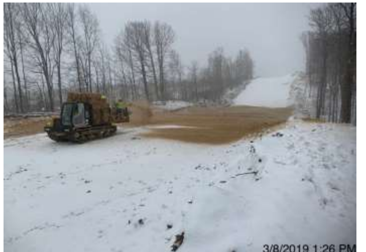
Spread 2-1 – Applying mulch over seed
