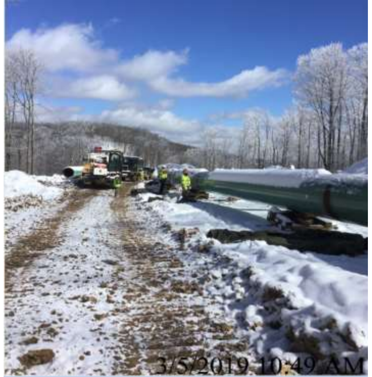
Spread 2-1 – Coating welds
