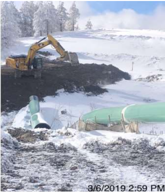
Spread 2A – Installing waterbars
