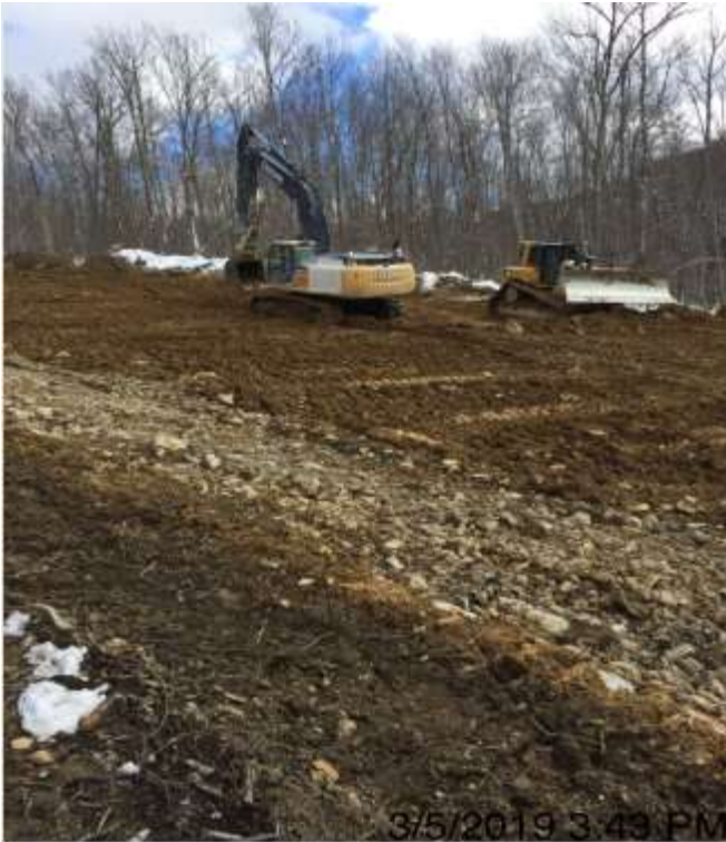
3/5/2019 3:43 PM Spread 2-1 – Installing water bars
