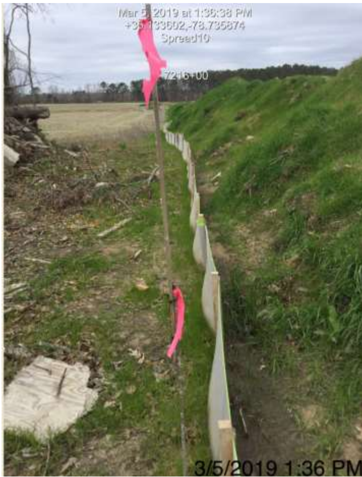
Spread 10 – Stabilized ROW
