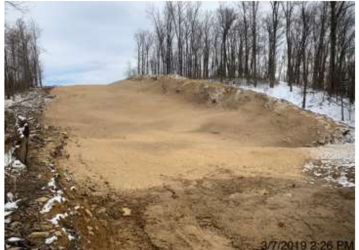
3/7/2019 2:26 PM Spread 2-1 – Stabilized ROW
