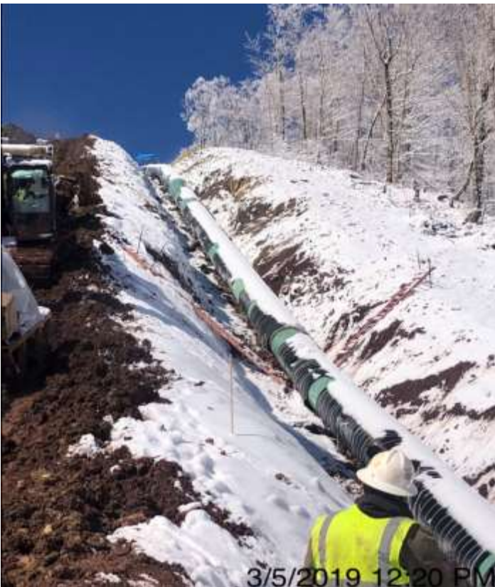
3/5/2019 12:20 PM Spread 2A – Tie in (top of the hill)
