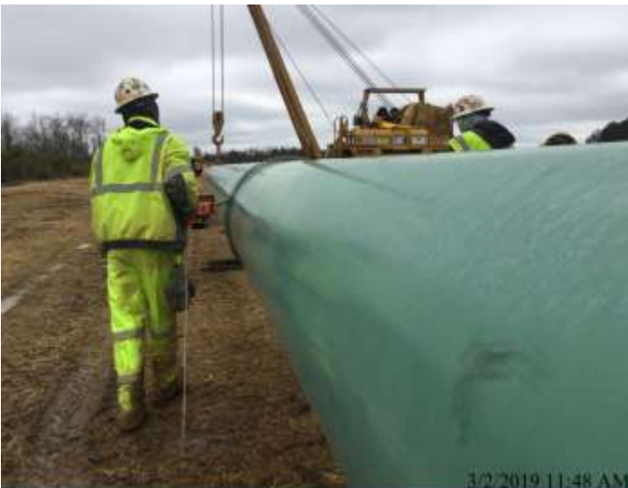
Spread 8 – Inspecting coating
