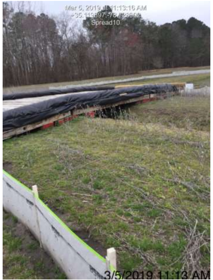
Spread 10 – Stabilized ROW
