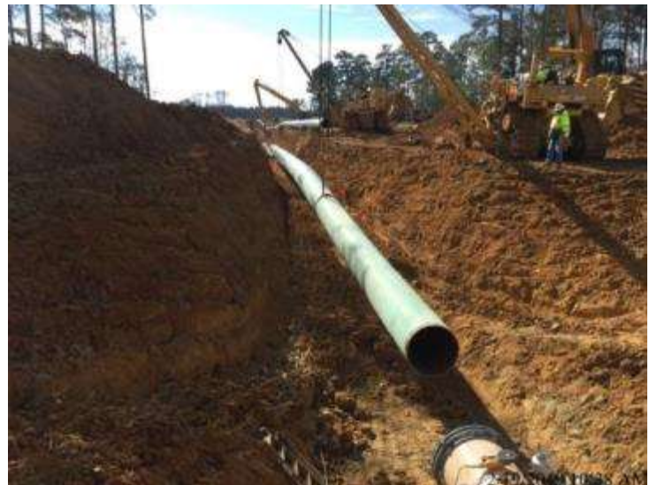
Spread 8 – Lowering in for tie-in weld
