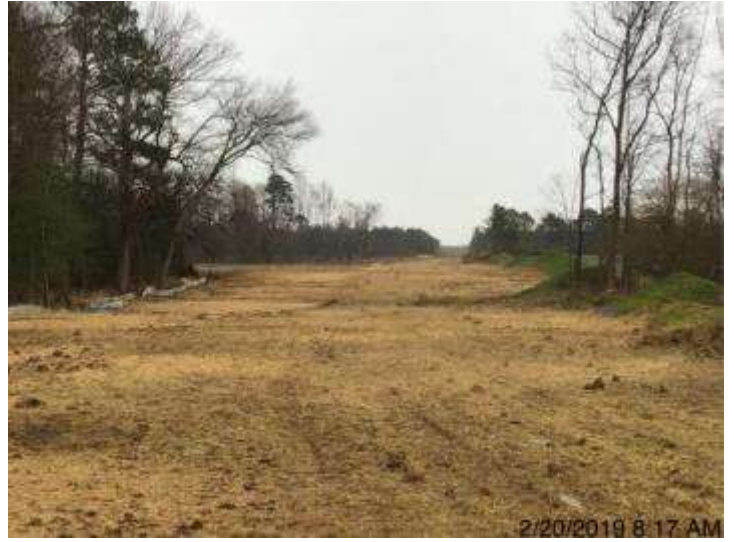
Spread 8 – Stabilized ROW
