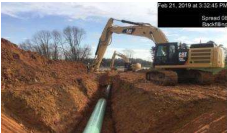
Spread 8 – Padding / Backfilling
