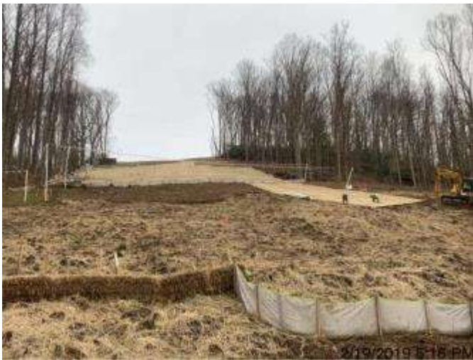
Spread 2-1 – Stabilized ROW
