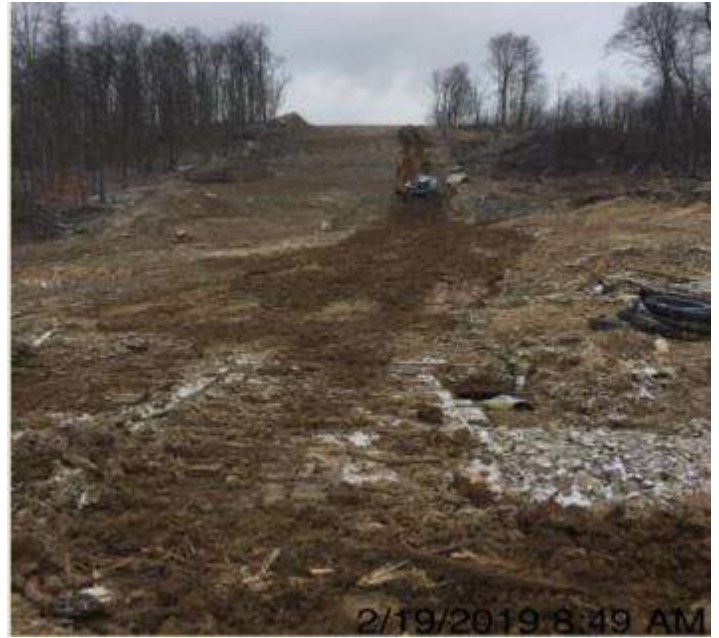
Spread 2-1 – Restoring grade
