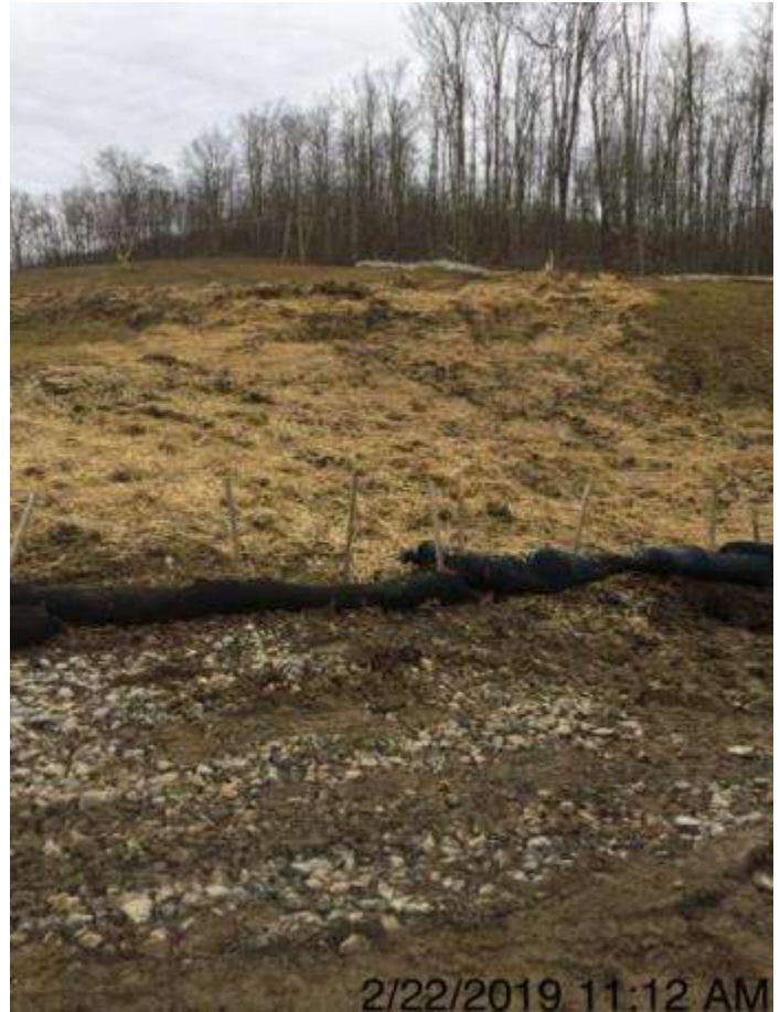
Spread 2A – Stabilized ROW
