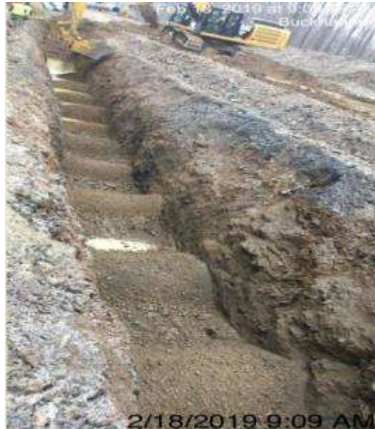
Spread 2-1 – Padding the ditch
