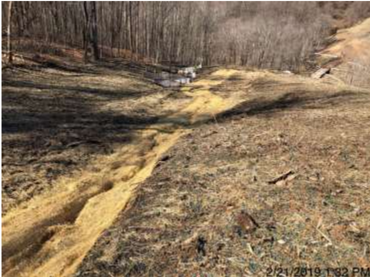
Spread 1-1 – Stabilized ROW
