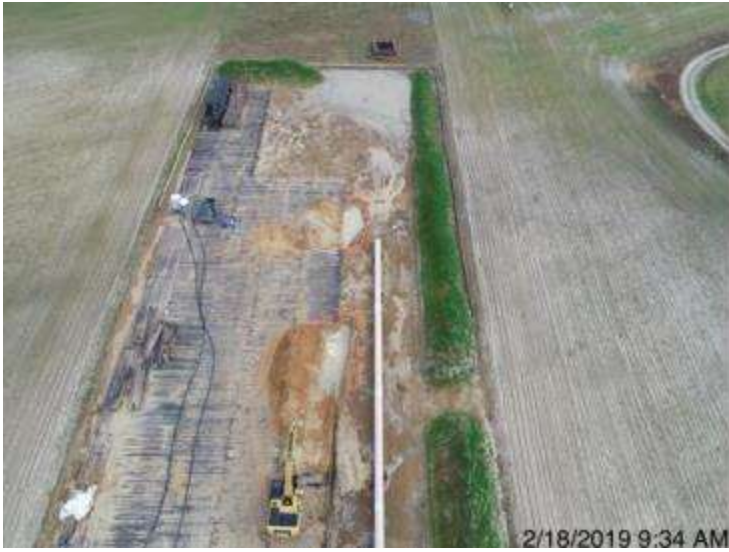
Spread 8 – HDD exit side
