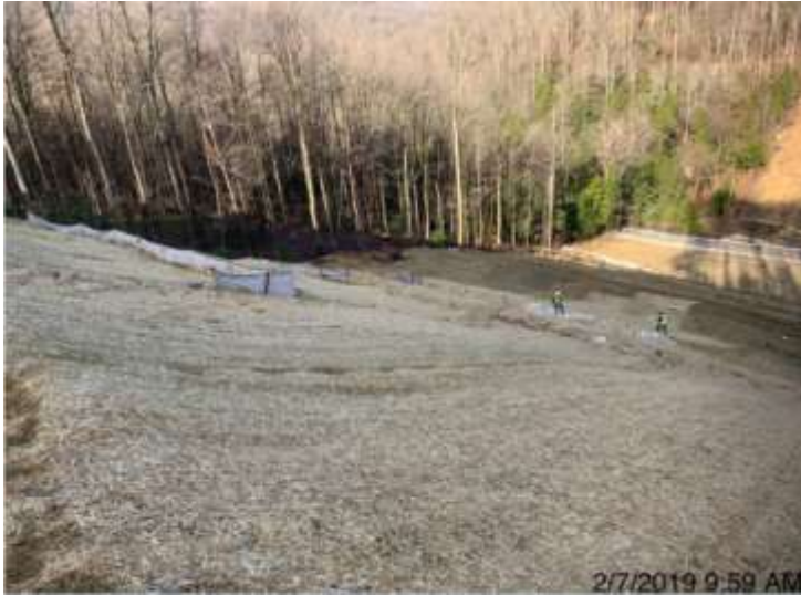
Spread 2-1 – Stabilizing the ROW
