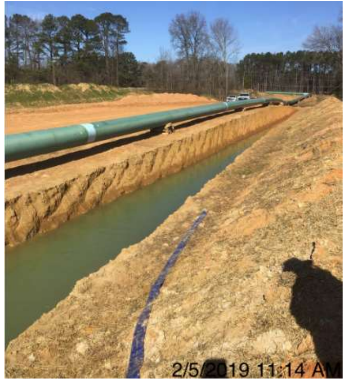
Spread 8 – Dewatering the ditch
