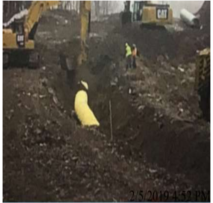
Spread 2A – Backfilling
