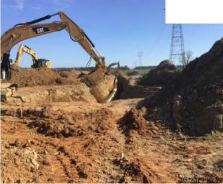
Spread 8 – Backfilling
