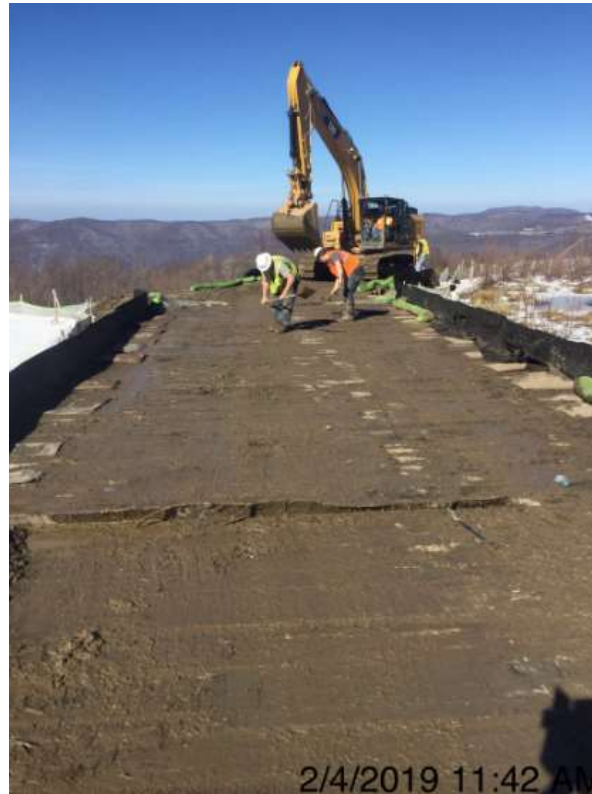
Spread 2A – Keeping bridges clean
