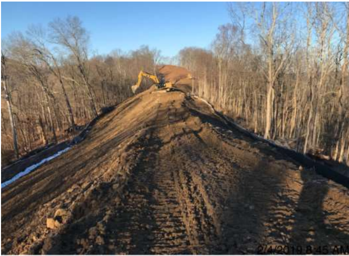
Spread 1-1 – ROW restoration
