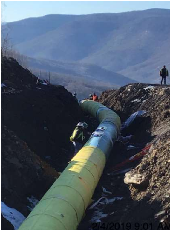
Spread 2A – Coating repair
