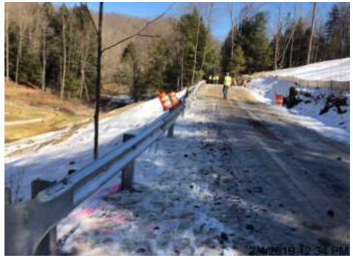
Spread 2-1 – Re-installing guard rails
