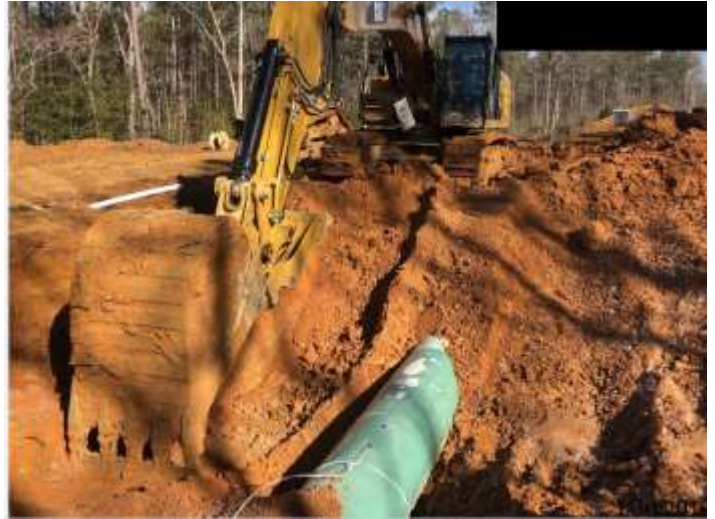
Spread 8 – Cathodic Protection Installation
