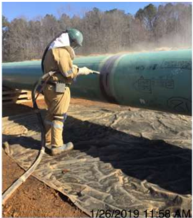
Spread 8 – Sandblasting A Weld
