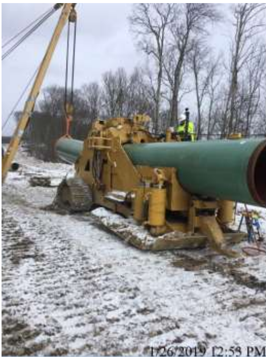
Spread 2-1 – Bending Pipe
