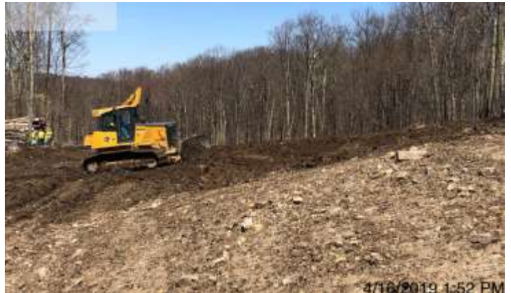
4/18/2019 1:52 PM Spread 2-1 – Cleaning up and drying the ROW
