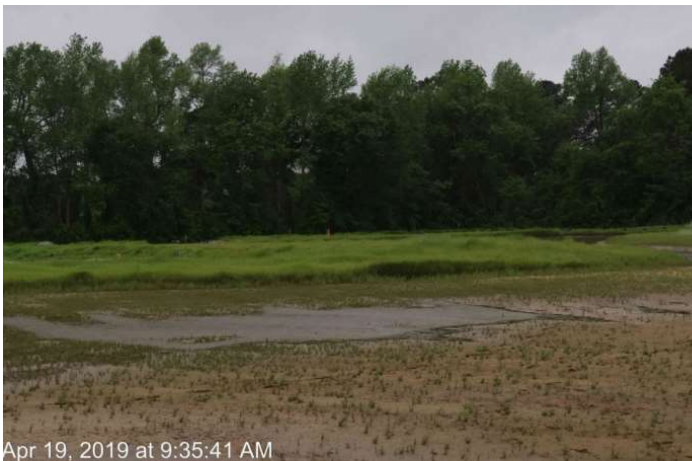
Spread 10 – Stabilized ROW after rain event
