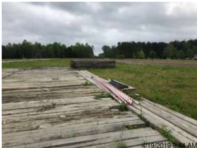
Spread 8 – Stabilized ROW
