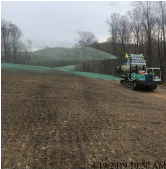
4/19/2019 10:50 AM Spread 2-1 – Hydroseeding
