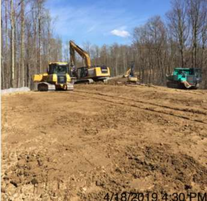
4/18/2019 4:30 PM Spread 2-1 – Preparing for seeding
