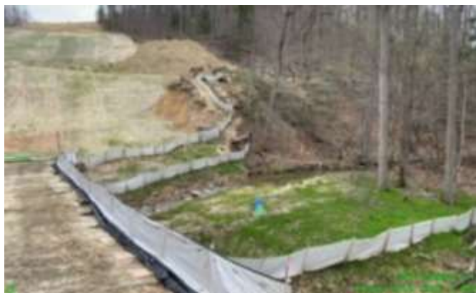
Spread 2A – Stabilized ROW
