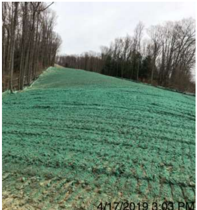
4/17/2019 3:03 PM Spread 2-1 – Hydroseeded ROW
