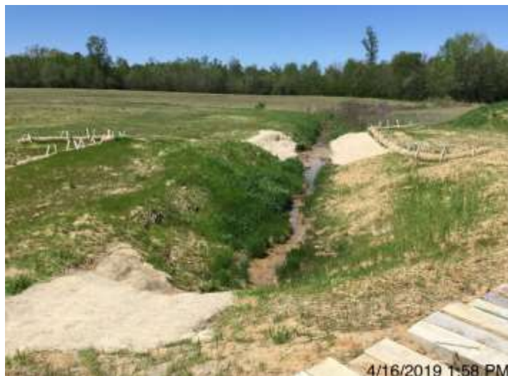
Spread 8 – Stabilized stream and ROW
