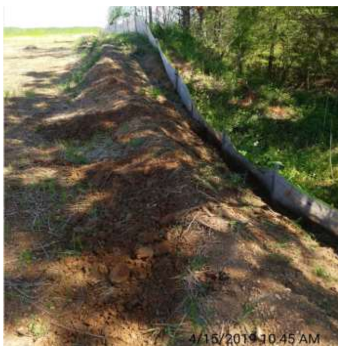
Spread 8 – ECD inspection
