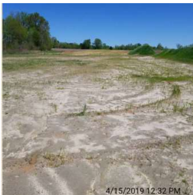
Spread 8 – Stabilized ROW
