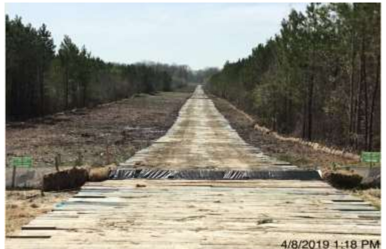
Spread 8 – Stabilized ROW
