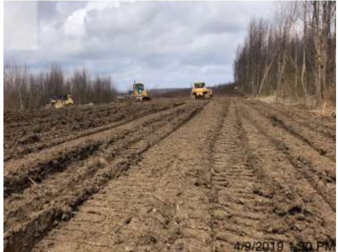
Spread 2-1 – Cleaning up and drying the ROW
