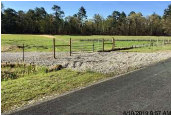
Spread 10 – Stabilized ROW
